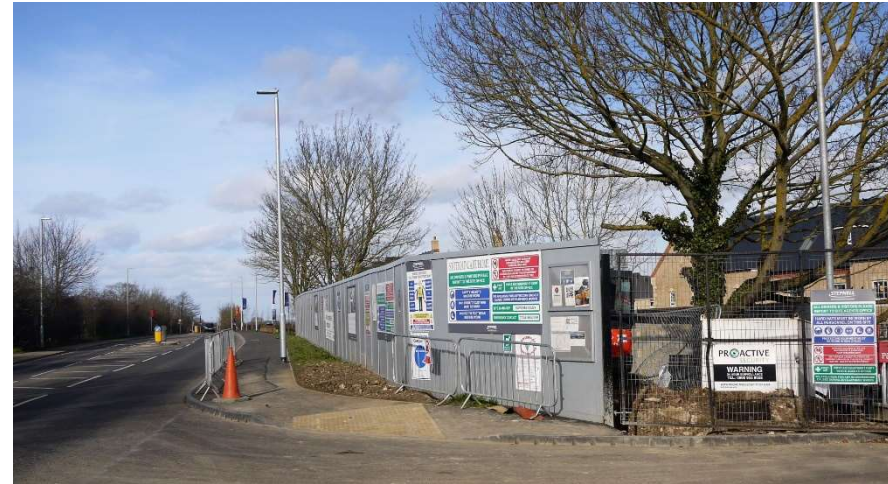
Construction site, Fairfield
