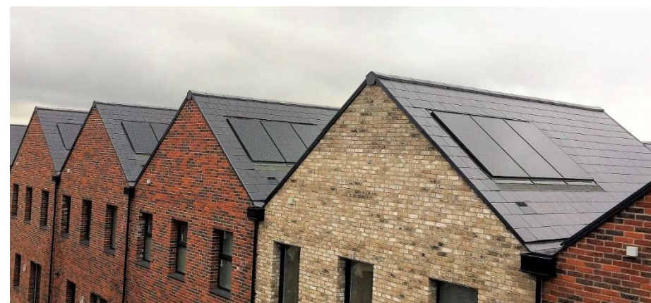
Solar photovoltaic panels, St Chads development, Tilbury (image © Photon Energy)
